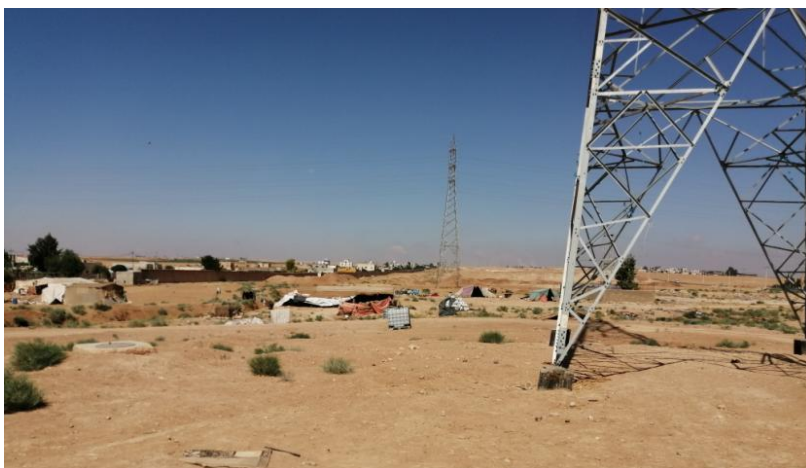
Figure 6.1: Bottom of the tower is not protected against climbing
